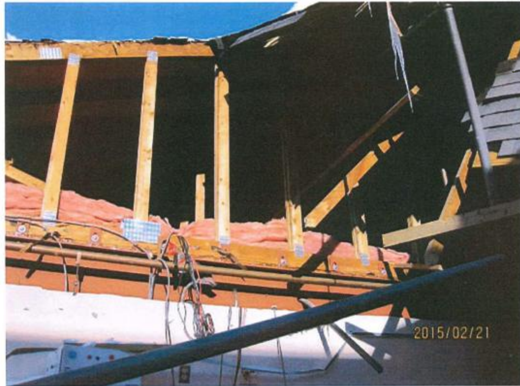
CENTRAL WING- SOUTH OF RIDGE-
